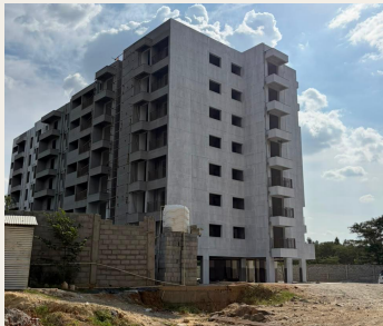
02 · WIDE BUILDING EXTERIOR IN PROGRESS
